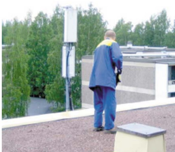
Figure 1. Working on a roof in front of a base station antenna.
